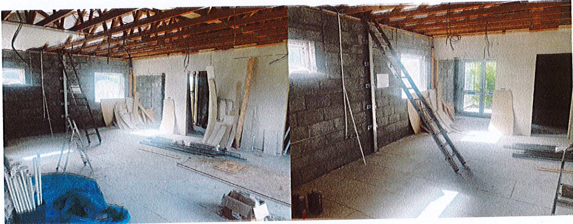
Figure 4 Latchbrook Community Centre showing first floor extension requiring completion
